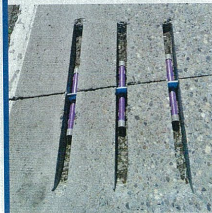
PHOTO: CTS CEMENT
