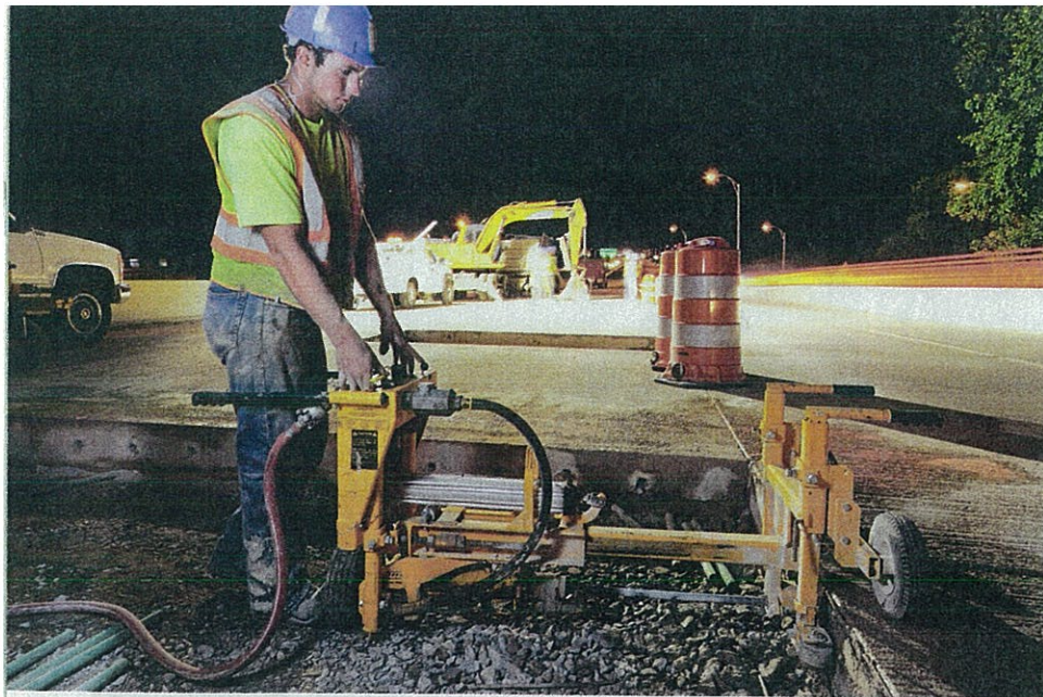
On-grade models operate from the subgrade level and are easy to position from one patch to the next. PHOTO: E-Z DRILL INC.
